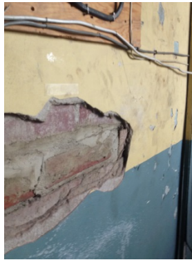
View plaster layers, NOT asbestos.
