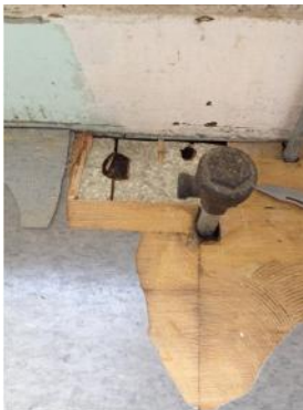
View of base layers of paint behind radiators
