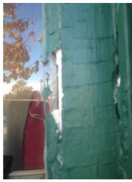
View of exterior green paint on Bldg 1
