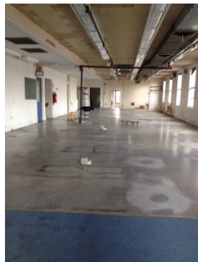
View of Building 2 2 nd level
