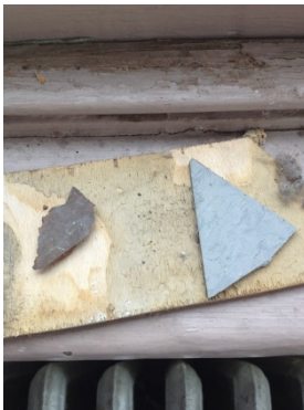
View of layers of flooring in Building 1 2 nd Floor (NOT asbestos)
