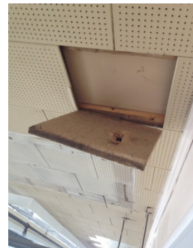
View of spline ceiling tiles NOT asbestos.
