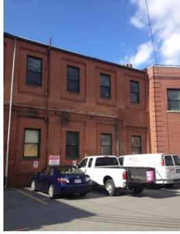
Building 2 Center portion
