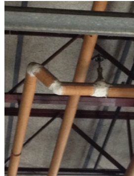
View of asbestos pipe joints Building 3
