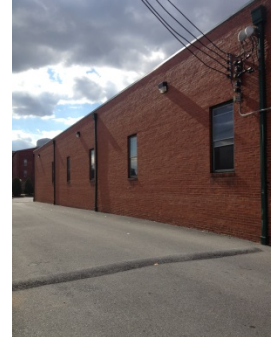
Building 3 Rear production area
