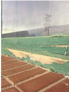
View of exterior green paint on Bldg 1
