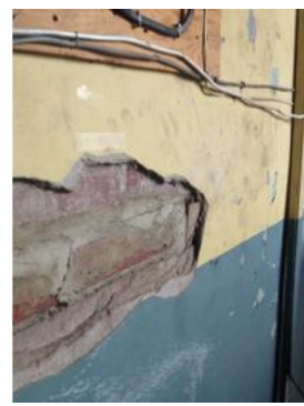
View blue and yellow paint in bldg 1 leading to basement
