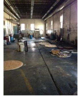
Building 3 Rear production area
