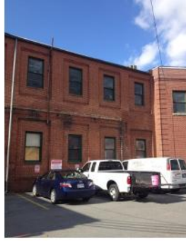
Building 2 Center portion
